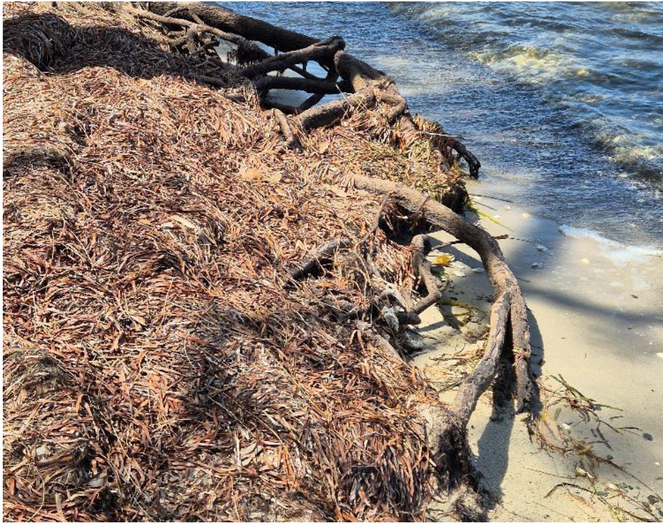
Figure 6-4 Site 3b, Reach 1- Undercutting of the foreshore exposing tree roots
