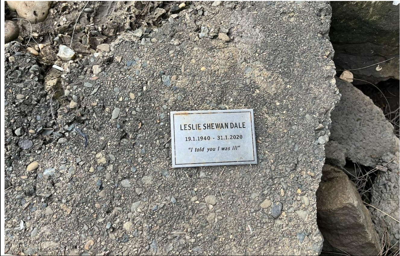
Photo 6: An example of a memorial plaque that may require relocation when concrete reinforcement is removed.
