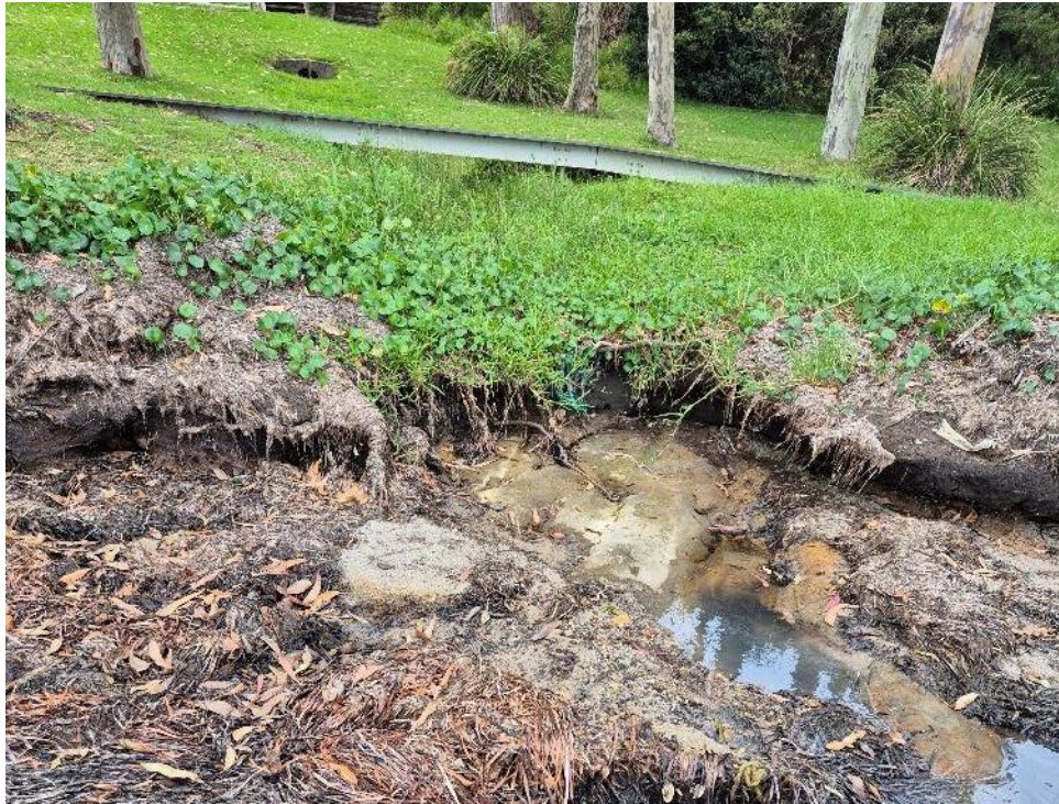
Figure 6-10 Headcut developing on a drainage line on the foreshore
