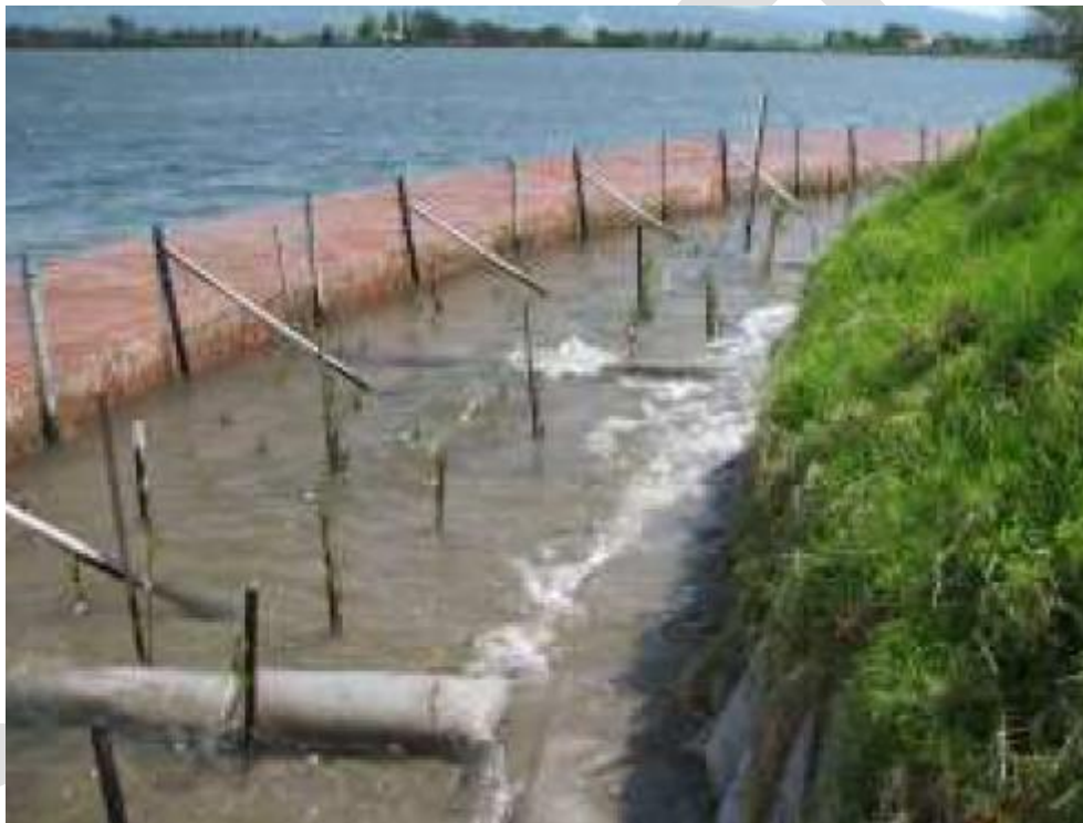
Figure 2-1 Sandbags and fencing used to shelter mangrove seedlings along Shoalhaven River (Source: Shoalhaven Riverwatch, 2013)
