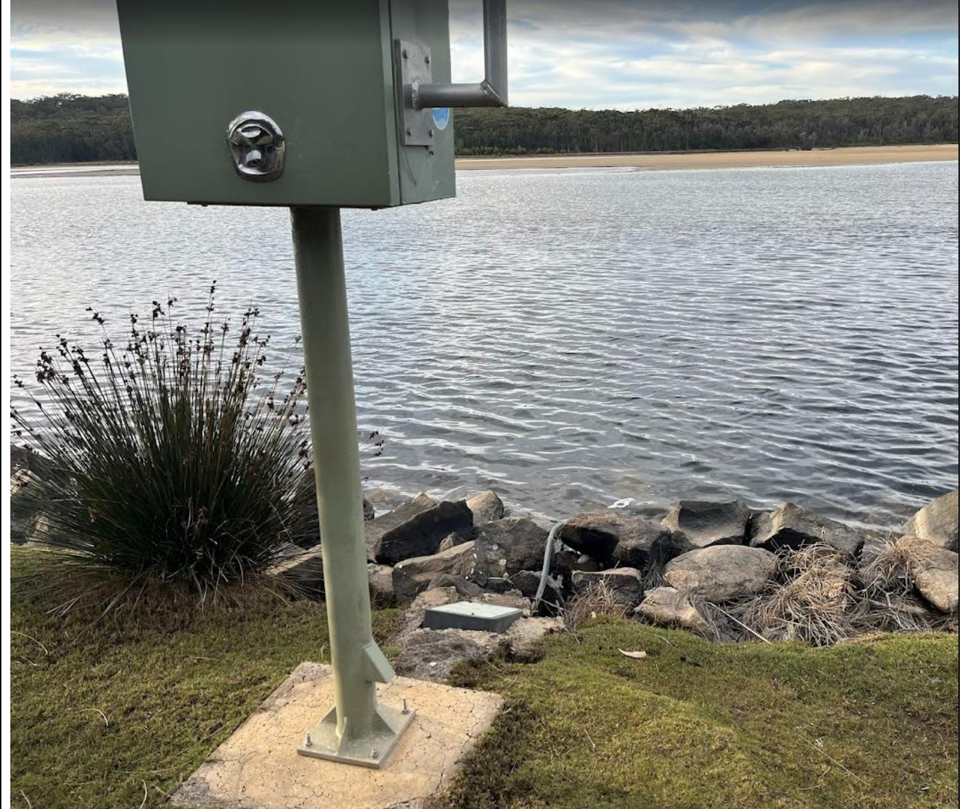
Photo 1: Manly Hydraulics monitoring equipment to be protected during rock placement works. Also showing invasive species Sharp Rush to the left.
