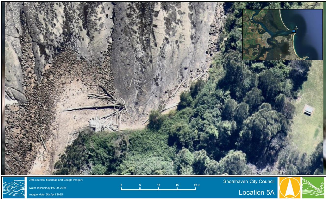
Figure 8-1 Site 5A location in Crookhaven Heads
