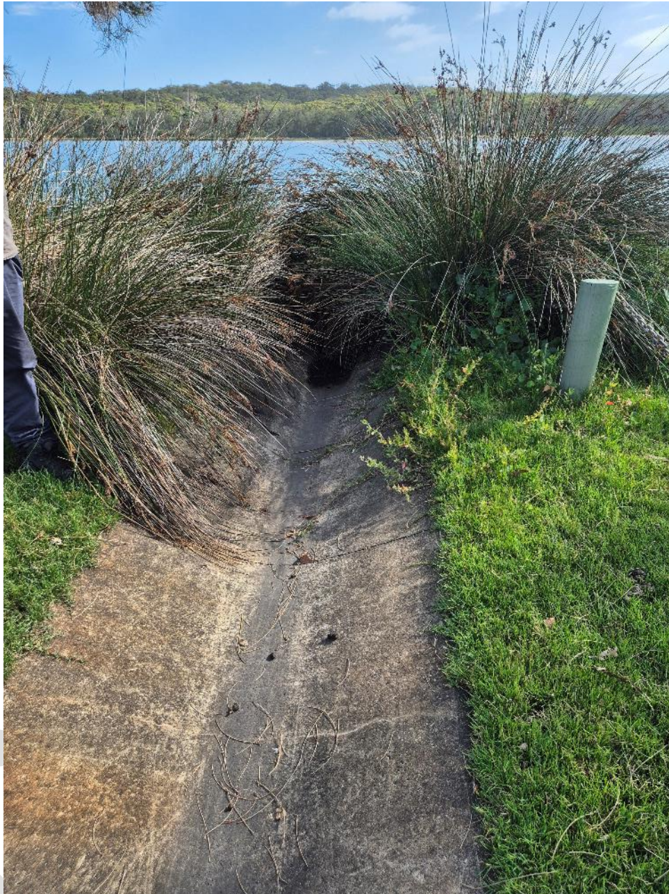
Figure 3-9 Spoon drain terminating at a stormwater pit.
