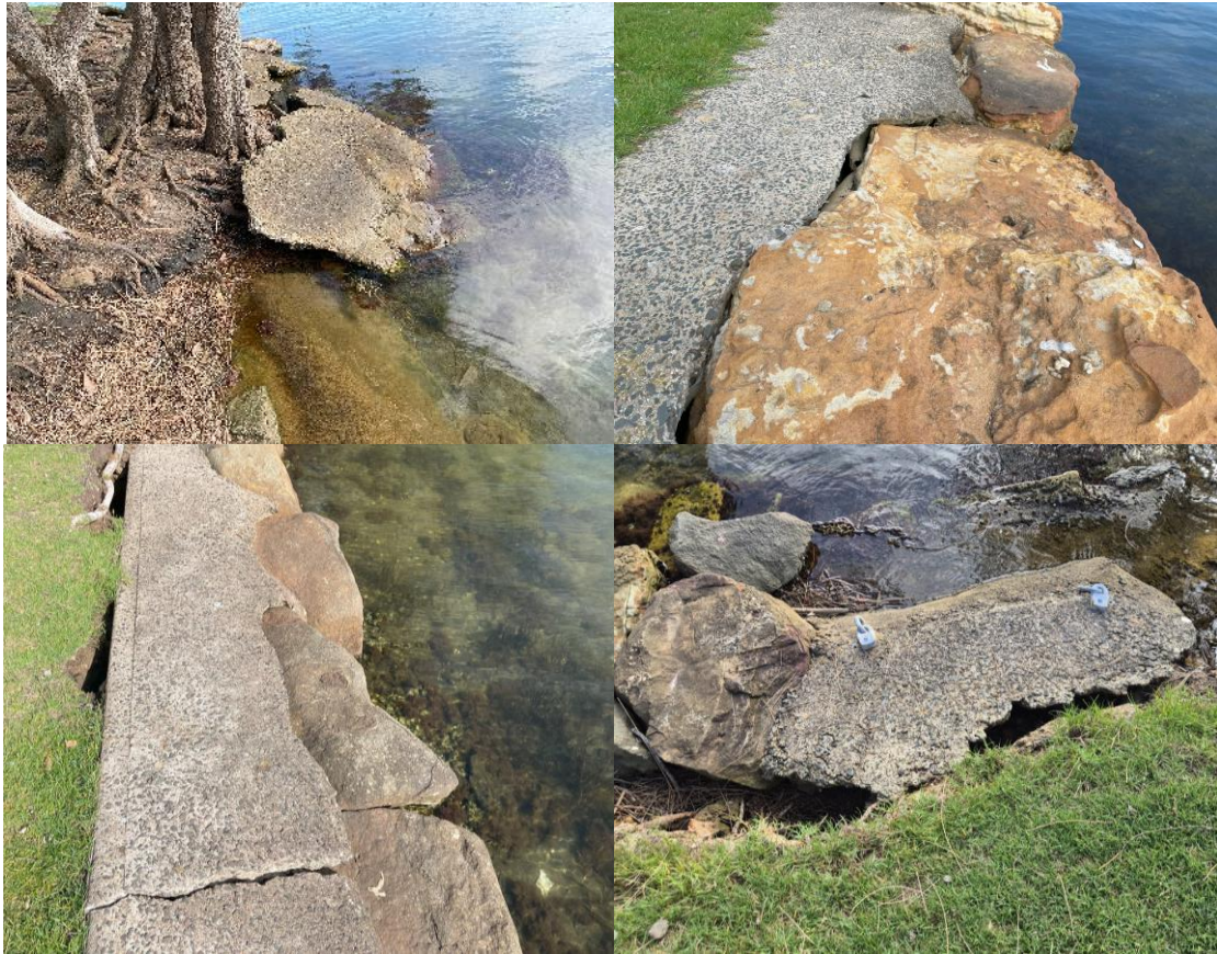
Figure 3-6 Examples of concrete reinforcement in poor conditions
